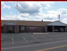
North Middleton Fire Company #1 310 North Middleton Road
