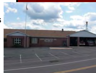
North Middleton Fire Company #1 310 North Middleton Road
